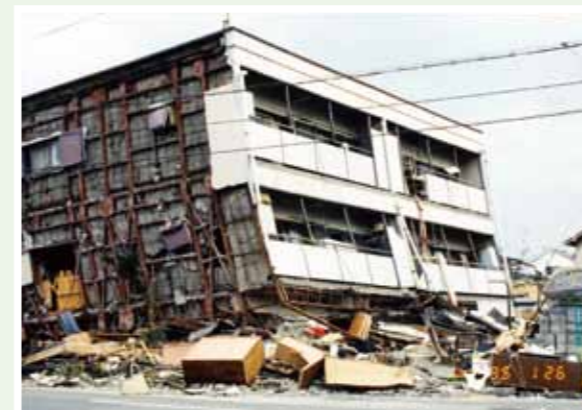
Collapsed Apartment Building (Great Hanshin Earthquake, January, 1995)
